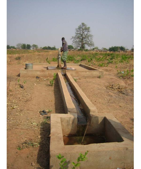
Deep Borehole Well with Lift Pump
