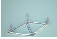
. First, lower members will be assembled together which make a base for the rest of structure.
